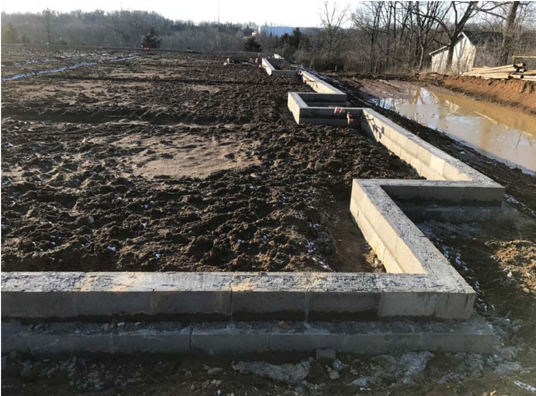
Masonry block foundation inplace on north end of building .
