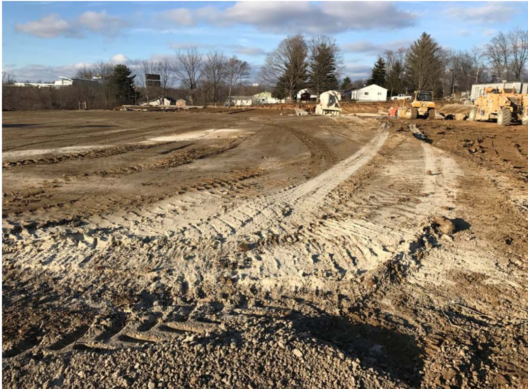
Newly compacted pad on the south end of the building.
