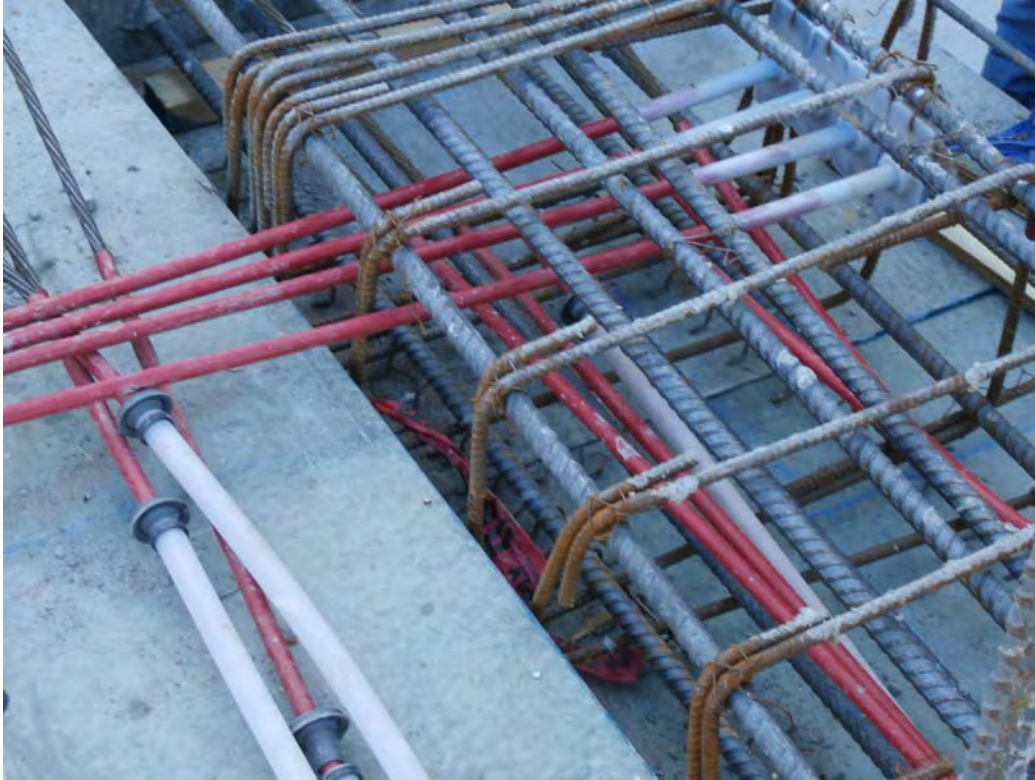
9. Installed PT cable
