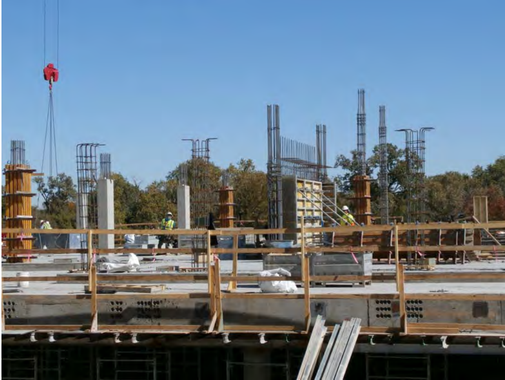
3. Shear wall forms on Level 3
