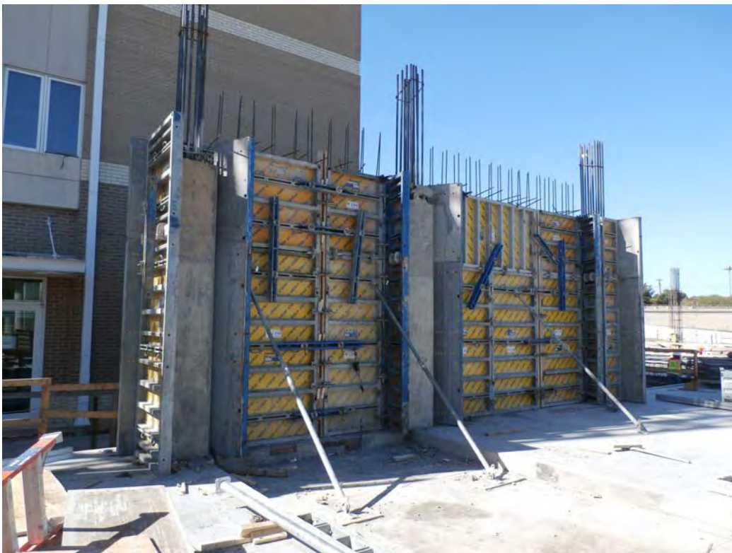
10. Shear wall formwork
