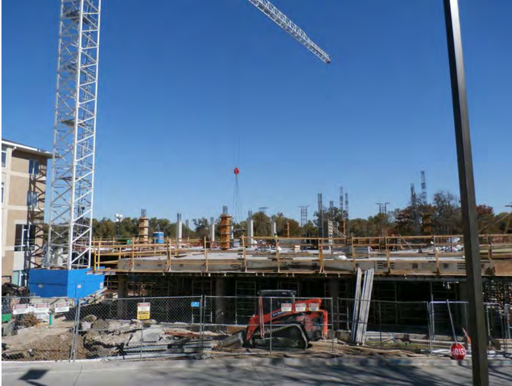
1. Level 3 column formwork
