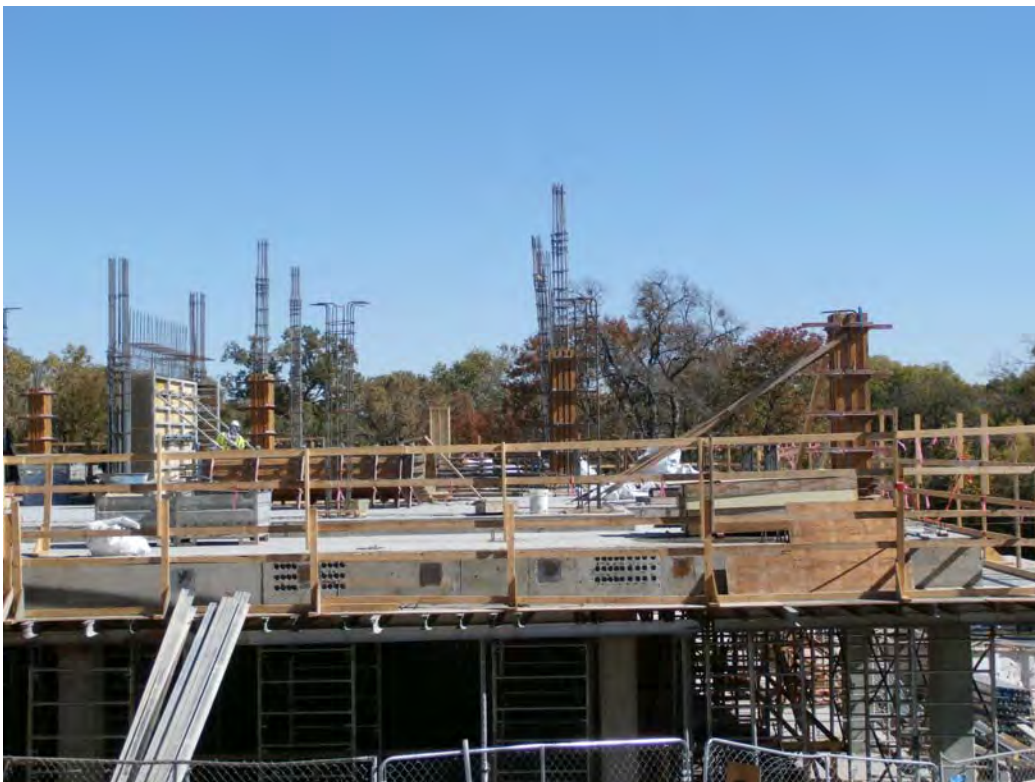
4. Work on Level 2 columns and shear wall
