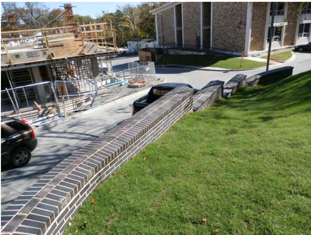
2. Completed brick radius wall coping
