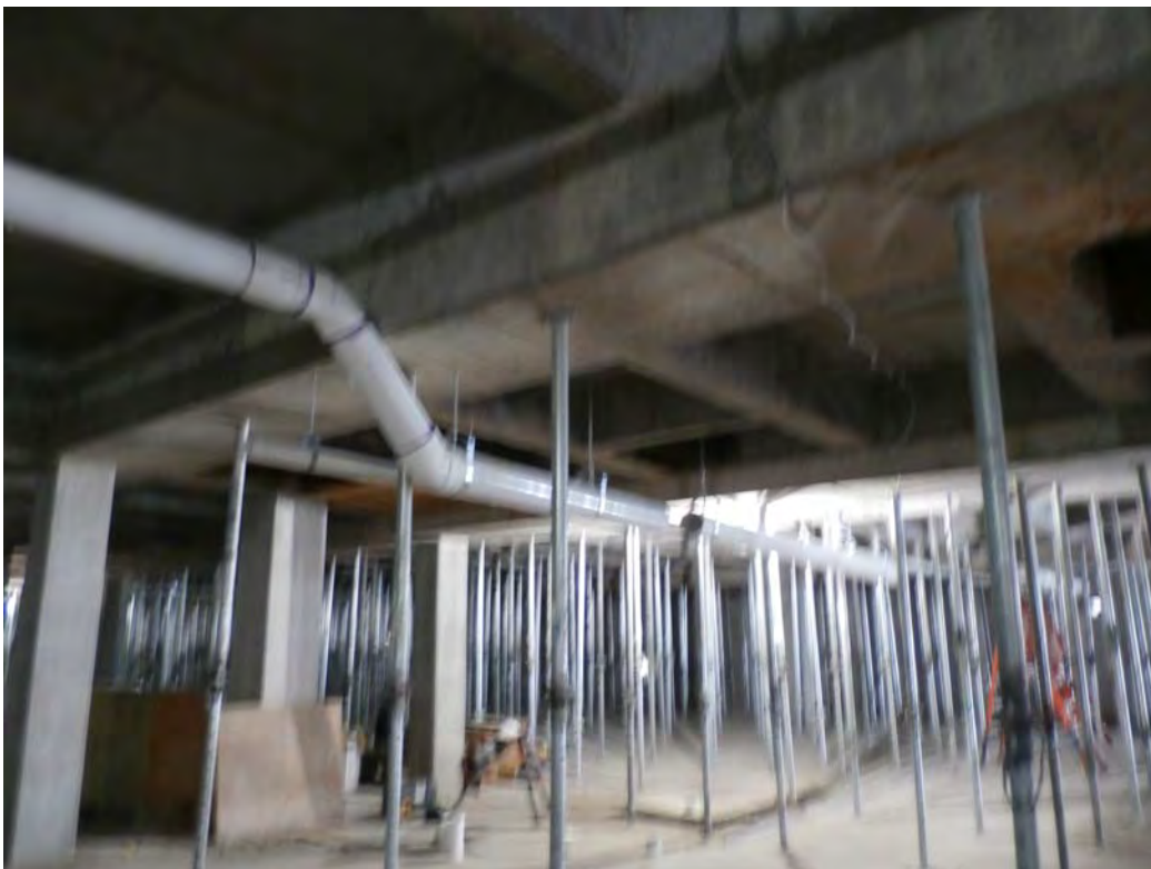
16. Garage installed drain lines
