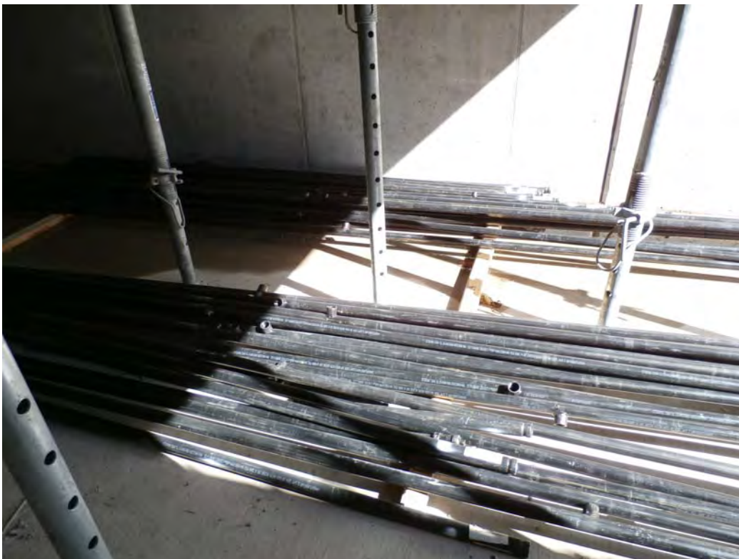
18. Garage staged sprinkler lines
