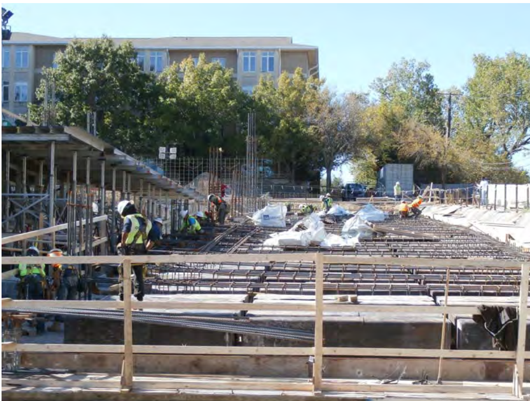
6. North deck preparation for concrete pour
