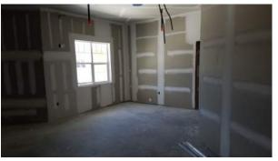
Figure 17-23 Interior framing and MEP rough in in various stages of completion.
