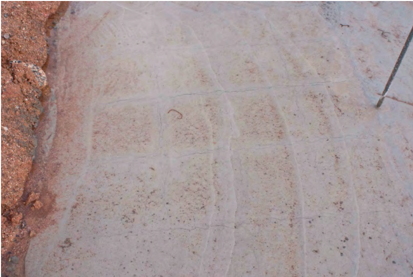
Figure 25 – Cracking in Footing – Building A
