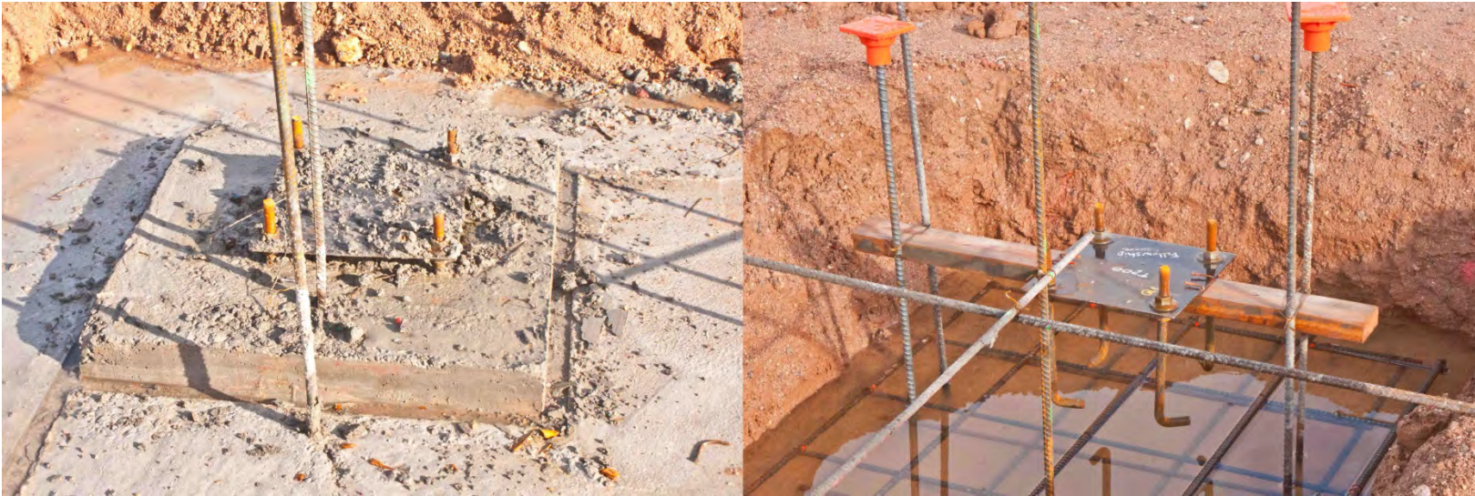
Figure 16 – Column footing with Anchor Bolts
