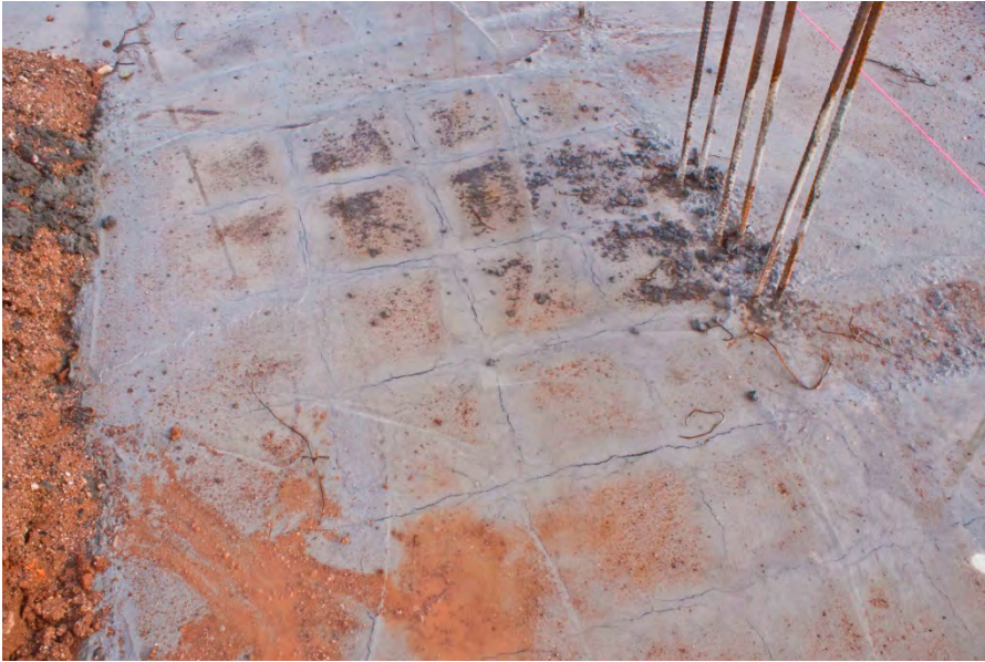
Figure 23 – Cracking in Footing – Building A
