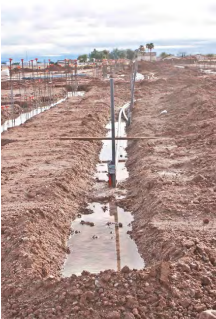
Figure 21 – Utility Trench at Building A
