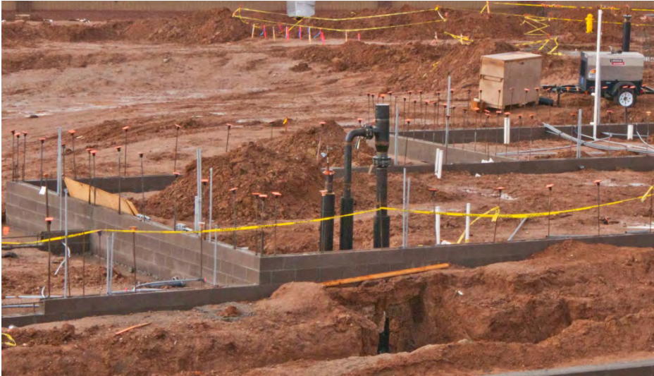
Figure 19 – Plumbing Piping at Central Plant
