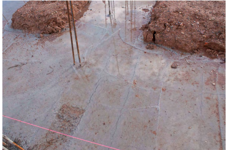
Figure 24 – Cracking in Footing – Building A
