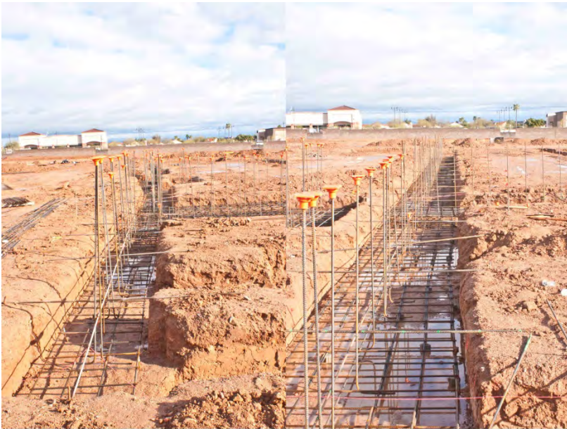
Figure 17 – Footing Trenches with Rebar
