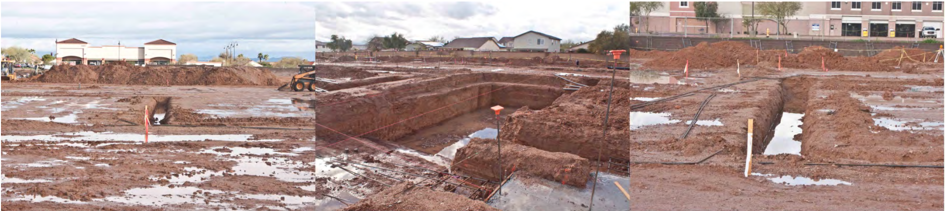
Figure 15 – Footing trenches
