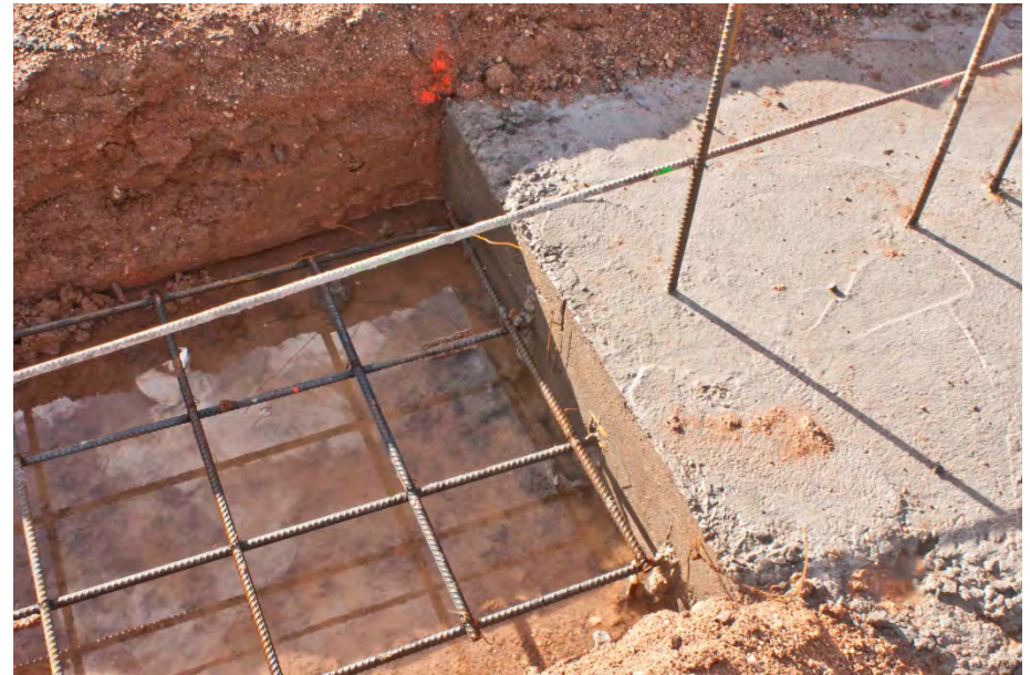
Figure 18 – Footing Cold Joint
