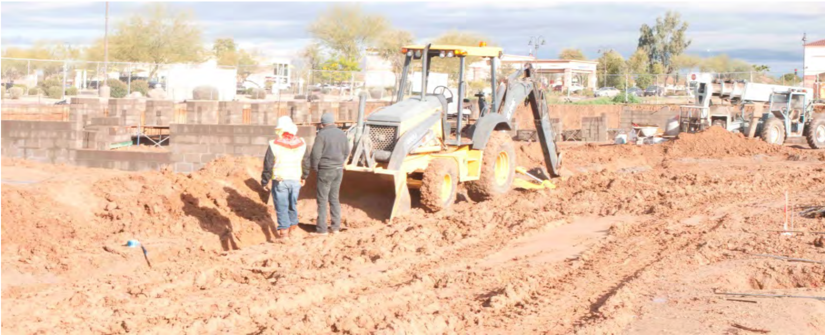
Figure 14 – Utility Trench Backfill
