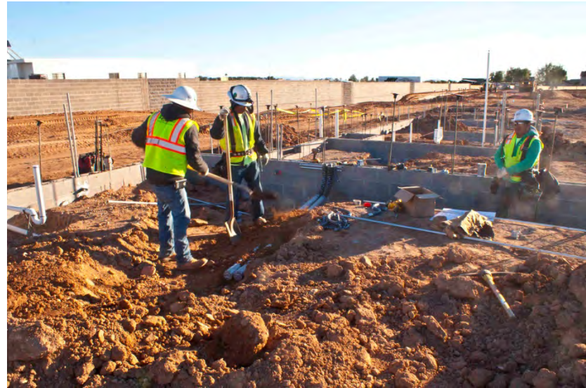
Figure 15 – Footing, Stem wall, under-slab utilities
