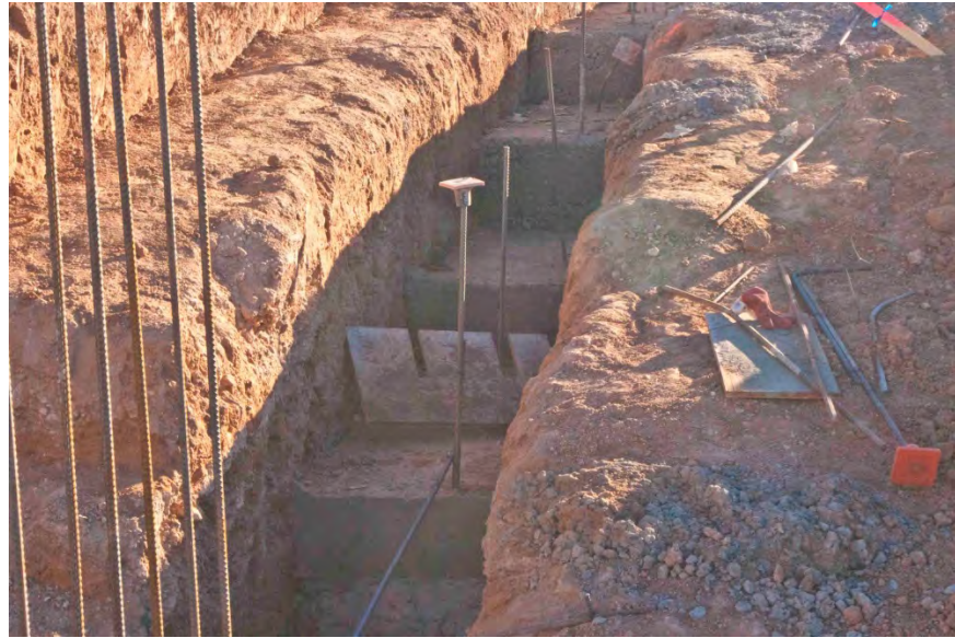
Figure 19 – Screen Wall Stepped Footing
