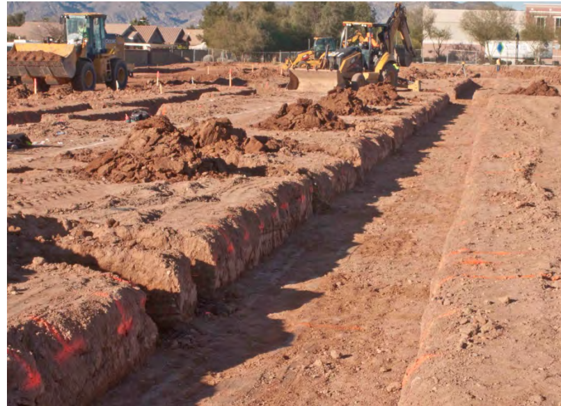
Figure 17 – Utility Trenching – Building A
