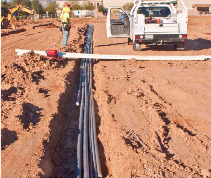
Figure 18 - Electrical Conduits - Building A
