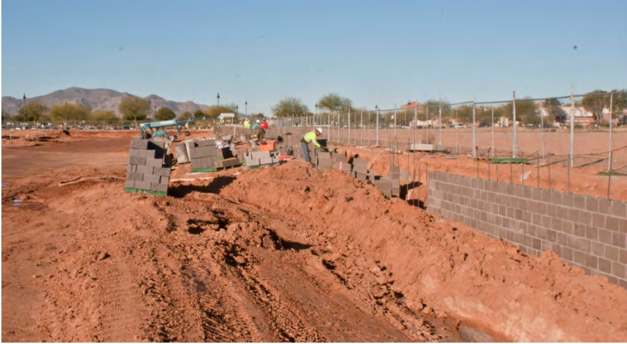
Figure 22 - Screen Wall Masonry Work
