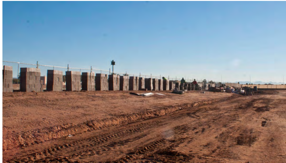
Figure 21 – Screen Wall Masonry Work
