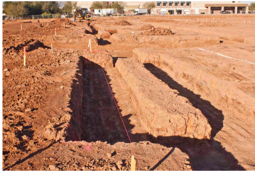
Figure 13 – Footing Trenches – Building A
