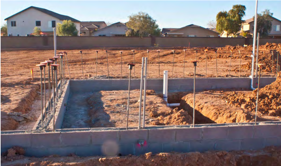
Figure 14 – Footing, Stem wall, under-slab utilities
