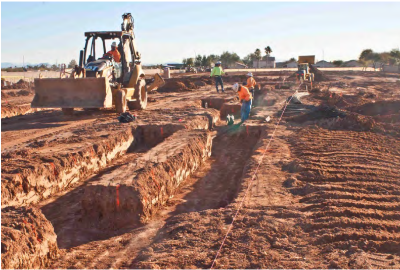
Figure 12 – Footing Trenches – Building A
