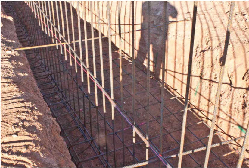
Figure 20 – Screen wall Footing
