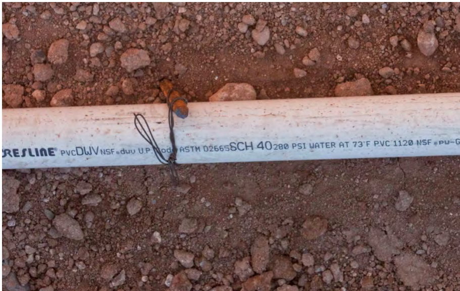
Figure 16 - Sewer Piping - Central Plant
